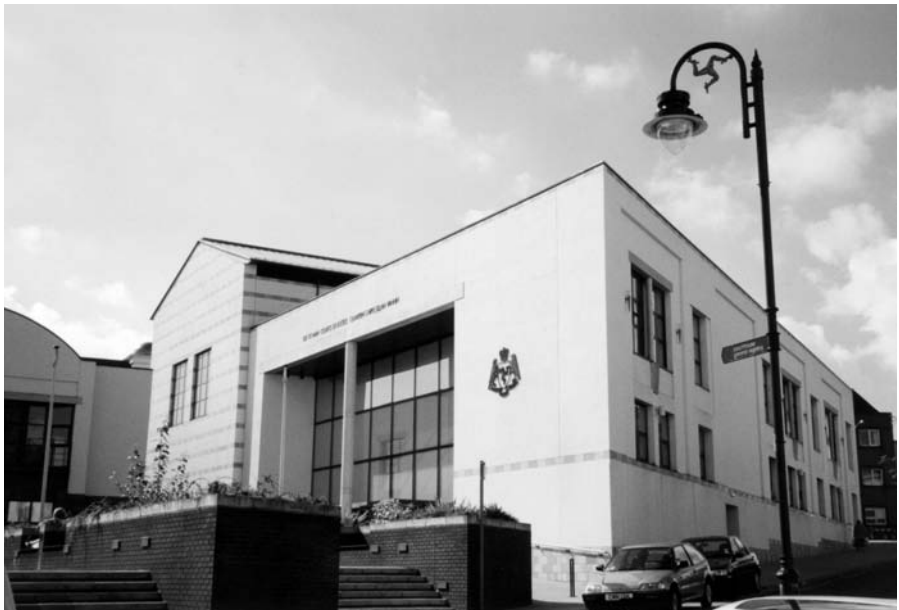
Isle of Man Courts of Justice, Douglas. The new courthouse and the adjacent registries building were built during the 1990s at a total cost of £10.4 million. They were officially opened by Chief Minister Gelling on 16 June 1997.
