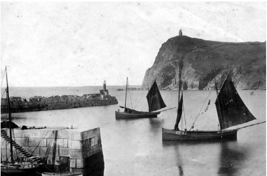
The Port Erin Breakwater, between completion in 1876 and destruction in 1884. The building and financing of the breakwater was the subject of prolonged negotiations between the UK and Manx authorities between 1861 and 1879.
