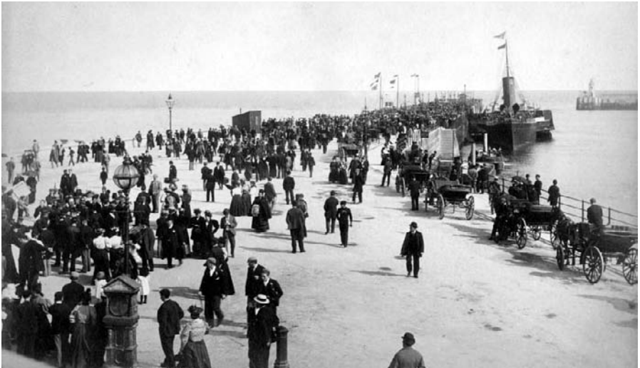
Victoria Pier, Douglas, between 1890 and 1900. One of the most important contributions made by government to the Manx economy between 1866 and 1900 was investment in harbour improvements. The Victoria Pier was opened by Loch in 1872, but was extended and modified between 1886 and 1890.
